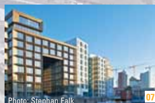
Office building at Rödingsmarkt Rödingsmarkt 16
